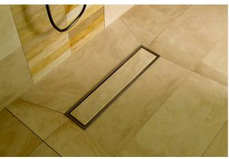
Linear drain—cover filled with tile.
